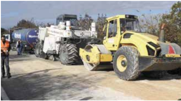
Figure 3. Recycling train on construction site
