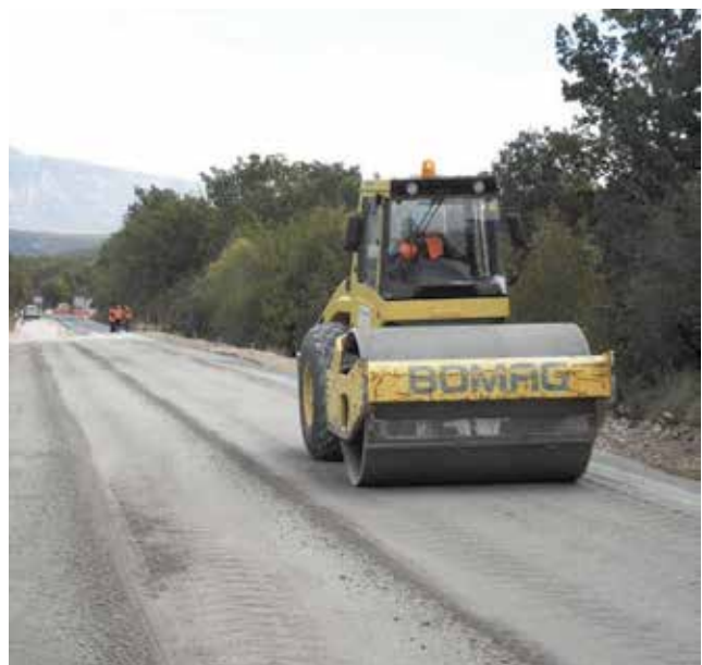
Figure 6. Recycled mix pre-compacting
