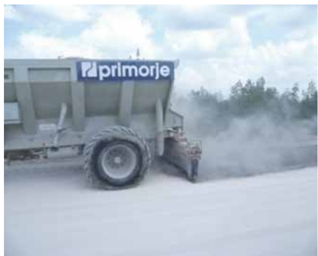
Figure 5. Spreading cement over the crushed aggregate
