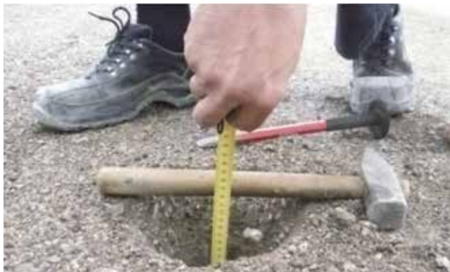
Figure 7. Checking thickness of the pavement base course
