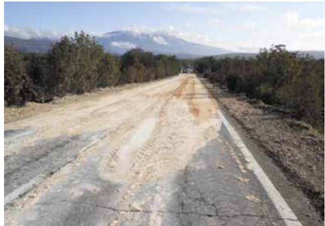
Figure 4. Spreading crushed aggregate over the existing pavement
